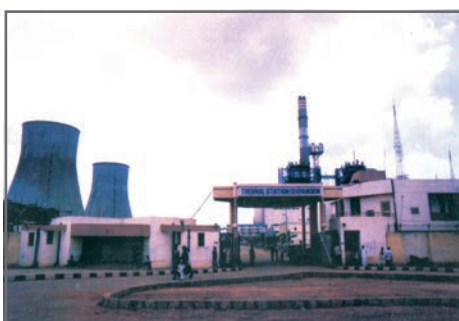
Fig 3.10: A view of a Thermal Power Station
