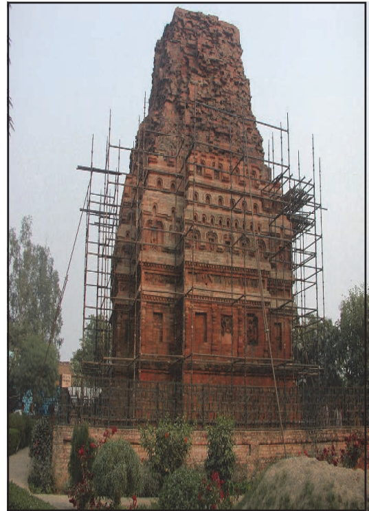
Pic. 9.3 Vishnu Temple in Bheetargaon, Kanpur (U.P.)
