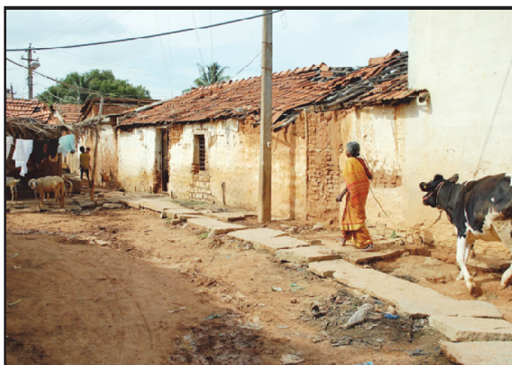
Pic. 3.4 Village with no proper facilities
